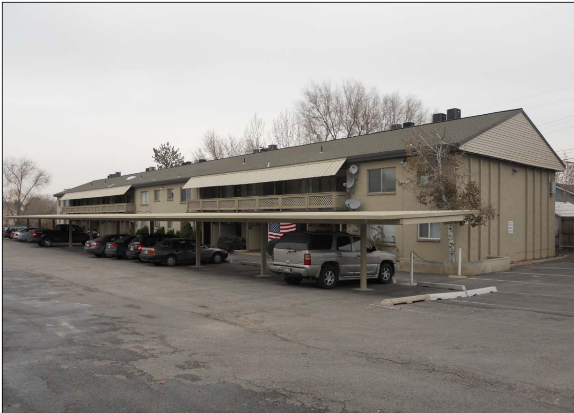
1946 S 900 E Rear (Interior of the Block "Boxcar" Multi-Unit Building)
